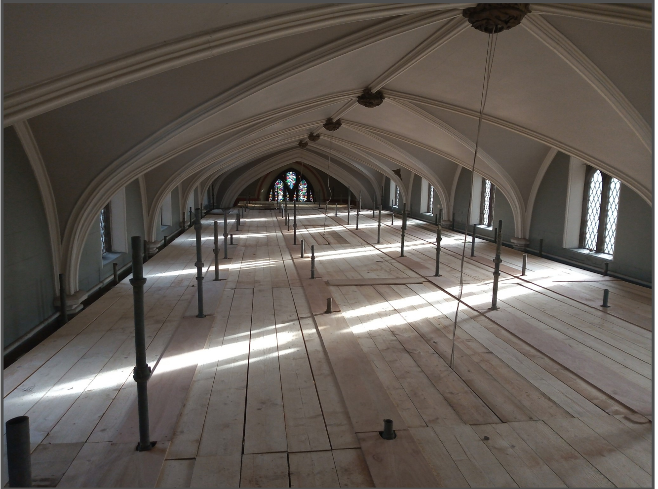
Above and left: photos of scaffolding in place.
